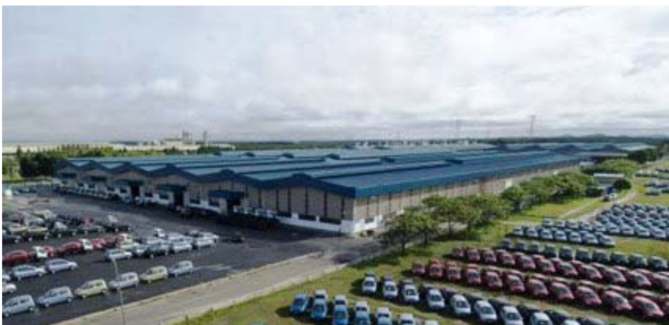
The BMW-Inokom assembly plant in Kulim.
