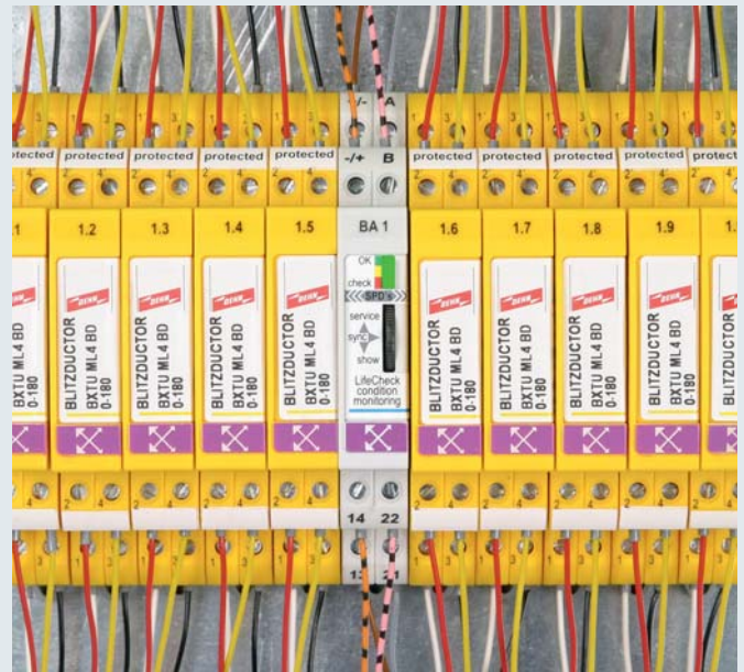
Installed DEHNrecord condition monitoring system
