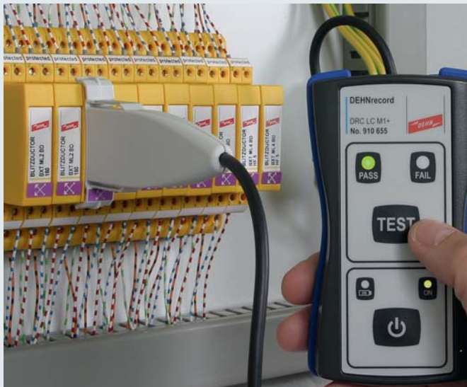
Testing a protection module via a hand-held device based on RFID technology (LifeCheck).
