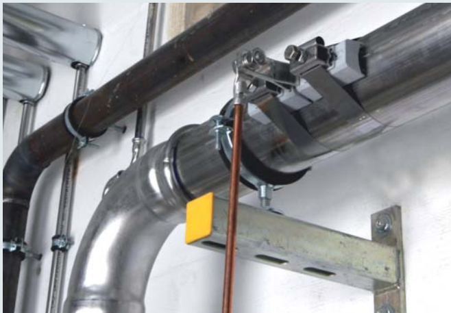
Installed at a StSt pipe
