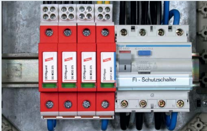
EMC-optimised series connection of lightning current and surge arresters according to IEC 60364-5-53 by means of STAK 2X16.
