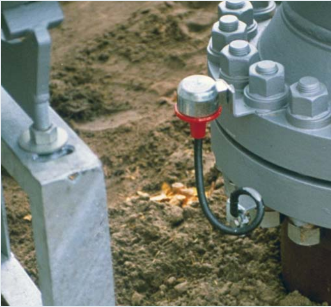
ATEX and IECEx-certified isolating spark gap for lightning equipotential bonding according to IEC/EN 62305 with flexible cable connection.
